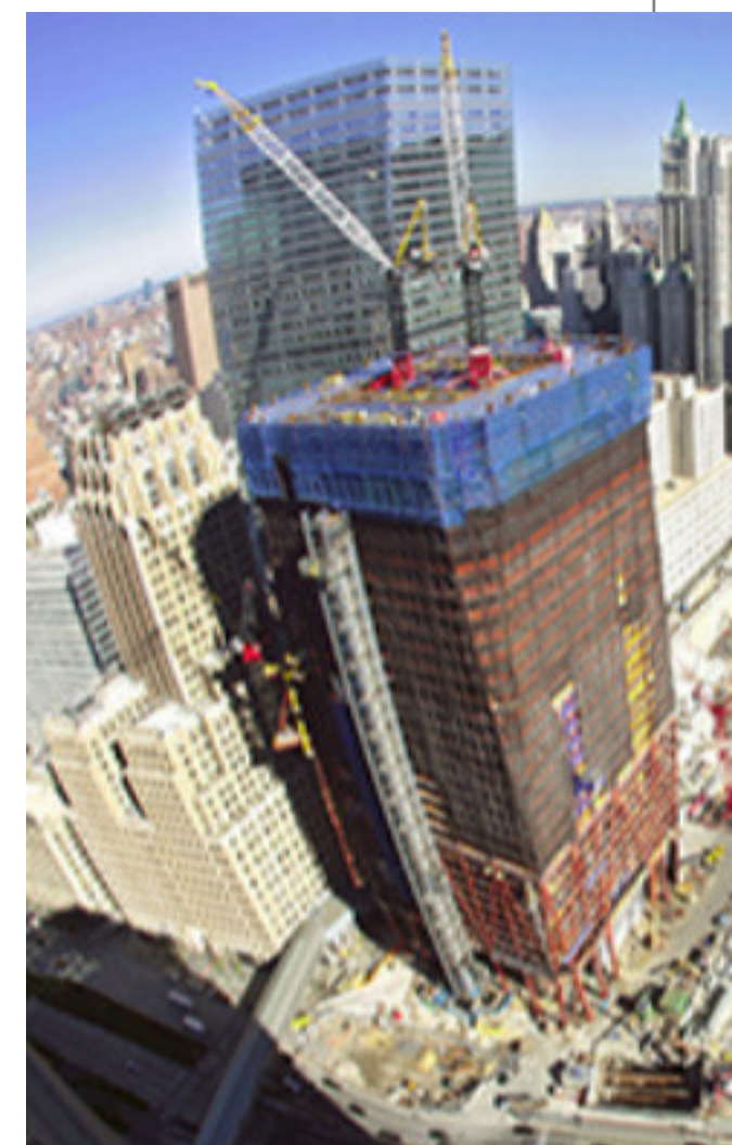
First time every part of the site is under construction. Foundation work began for World Trade Center. First time every part of the site is under construction.
